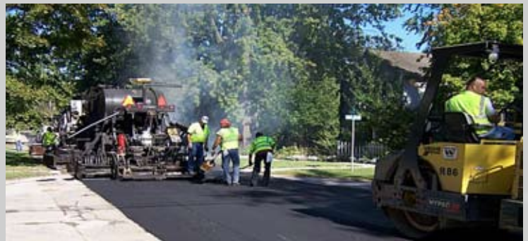
Hot-In-Place finished product.
