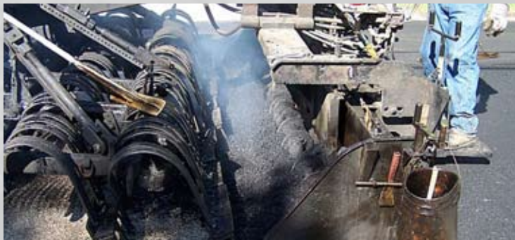
Scarifiers and an auger pulled by the second truck prepare the aggregate to be compacted.
