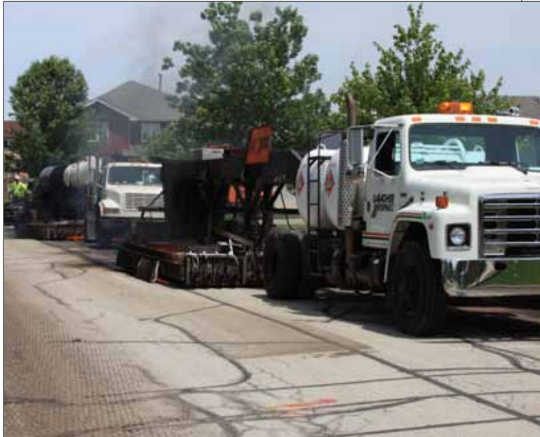
A combination of hot-in-place recycling (HIR) and thin overlays will last longer, says a Michigan county official.
