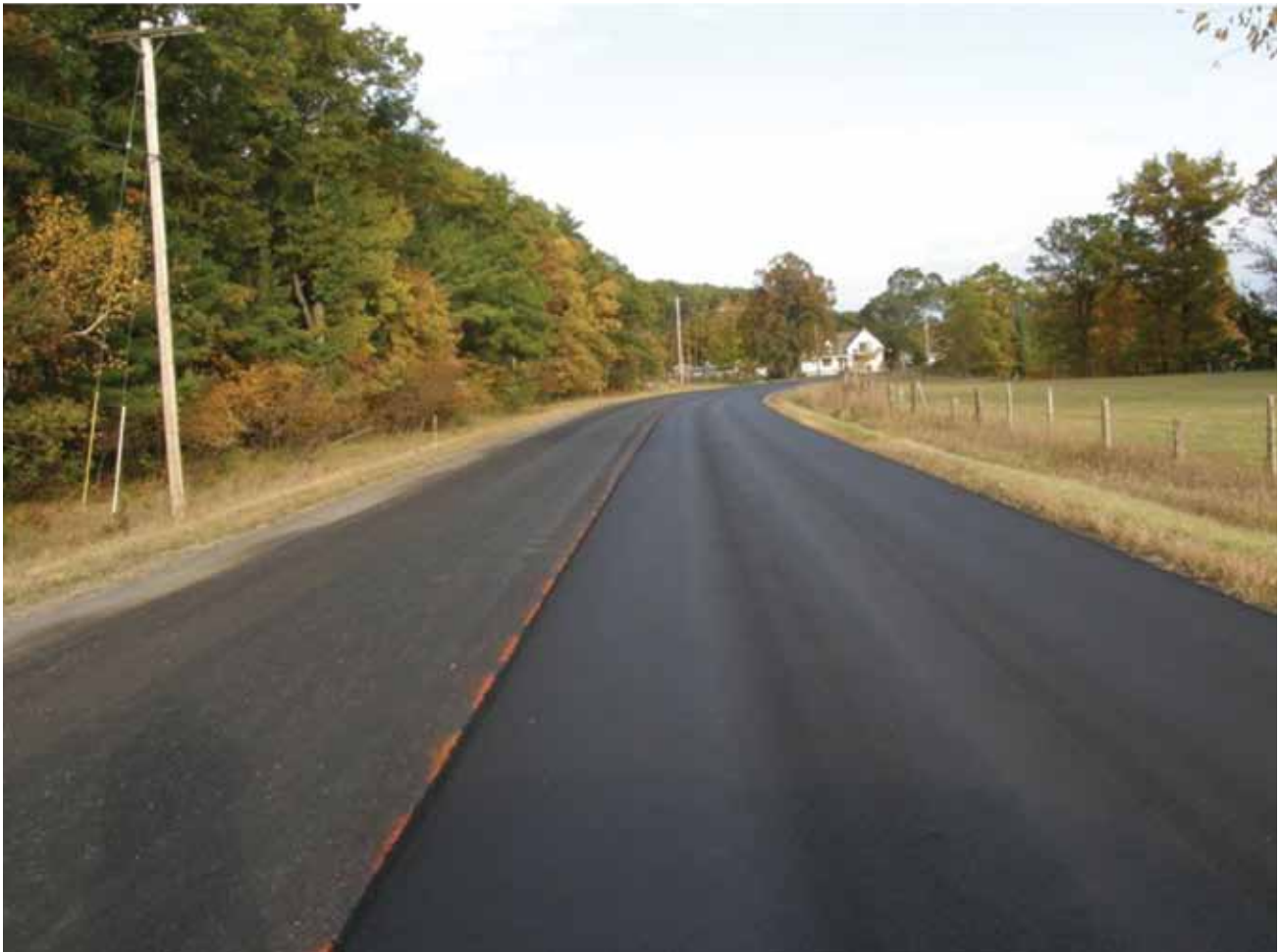
The ultra thin mix specified (right lane) for the project is a commercial ADT (average daily traffic) design requiring a PG 64-28 polymer modified binder. The left lane illustrates how the Hot In-Place process rejuvenates an aged pavement.
