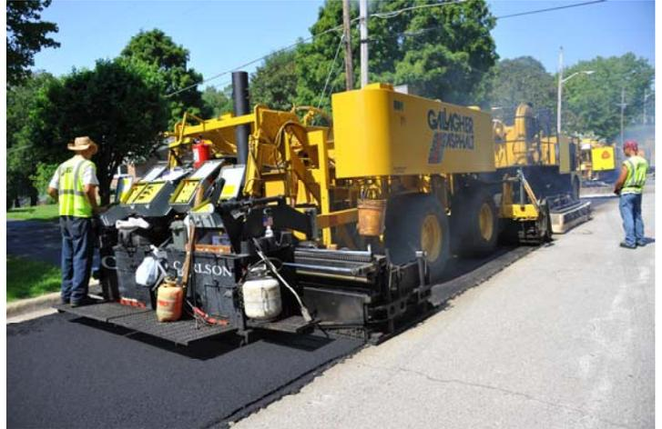
involves two sets of equipment – a pre-heater and a heater/scarifier. Combined, the two units are less than 120 feet in length. The first unit pre-heats the existing asphalt pavement to about 200 degrees. Immediately following, the heater/scarifier continues to heat the pavement to about 320 degrees while scarifying to a depth of typically 1.5 inches. After scarified, the pavement
